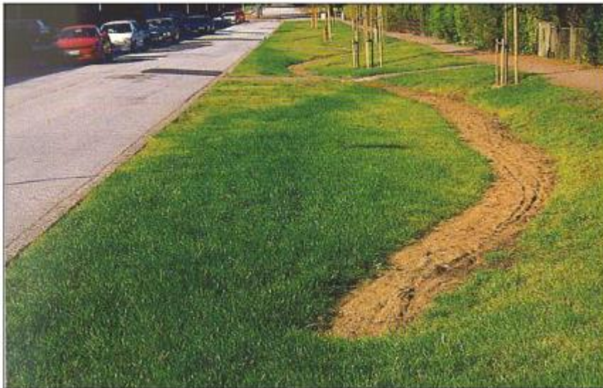
Figur 10 Svackdike (Ref: Peter Stahre)
